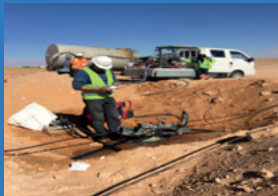
Blowing 135 km FOC at CPF Project
